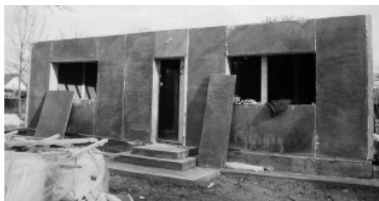
Wall panel of glass fiber reinforced mineral matrix[2]
