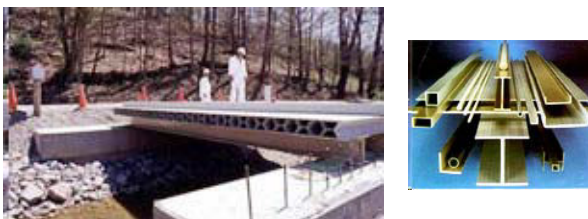
FiberlineBridge, using the pultruded profiles [1]
